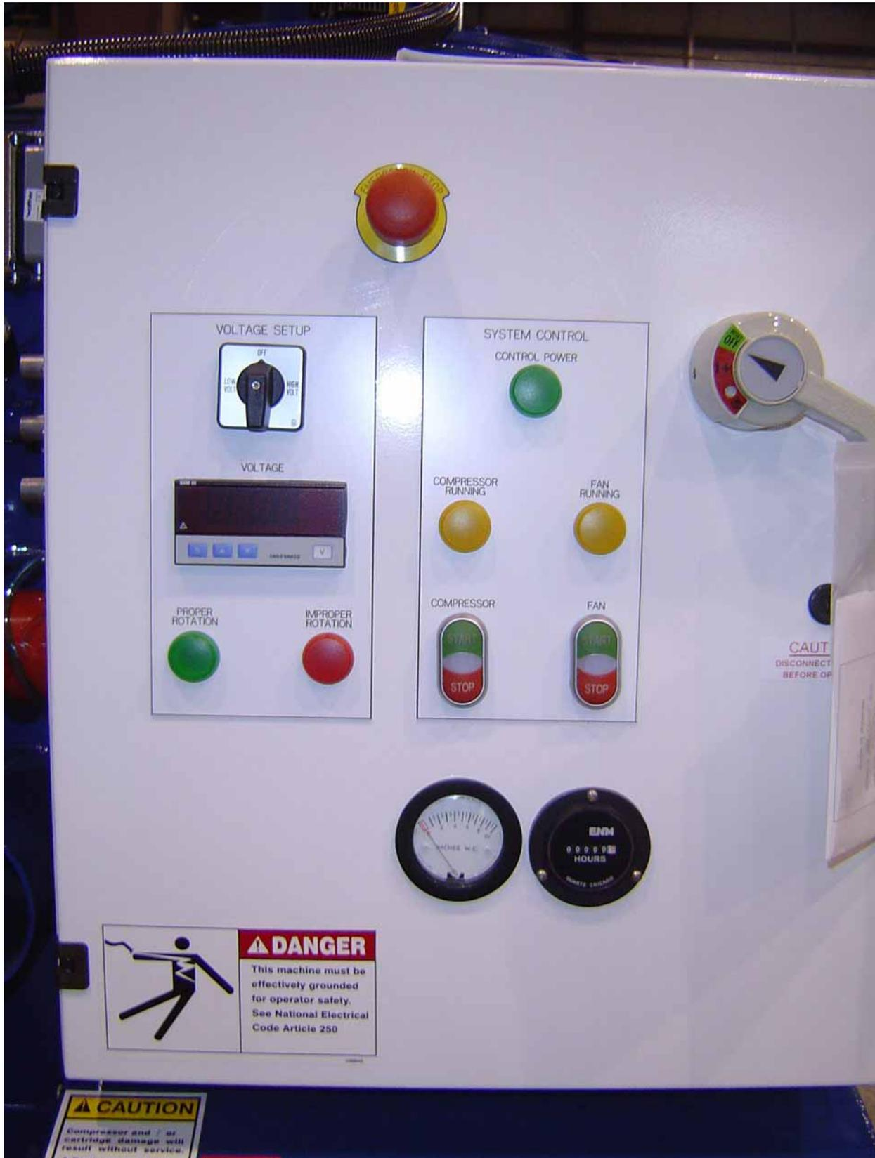
Fuseless Coordinated Motor and Circuit Protection – This control system was designed to comply with the National Electric Code as a “multi-motor and other loads” branch circuit. The control elements in this system have minimum withstand rating of 50 kA when the branch circuit providing power is protected with a listed fuse or breaker of equal or greater rating.
